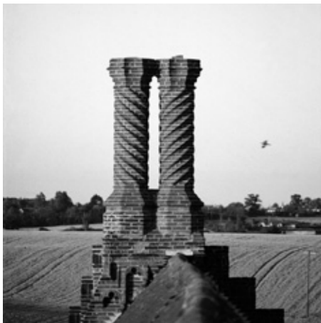
Cheminées Tudor | Tudor Chimneys, Loyer Marney Tower, Essex, Royaume-Uni | United Kingdom
